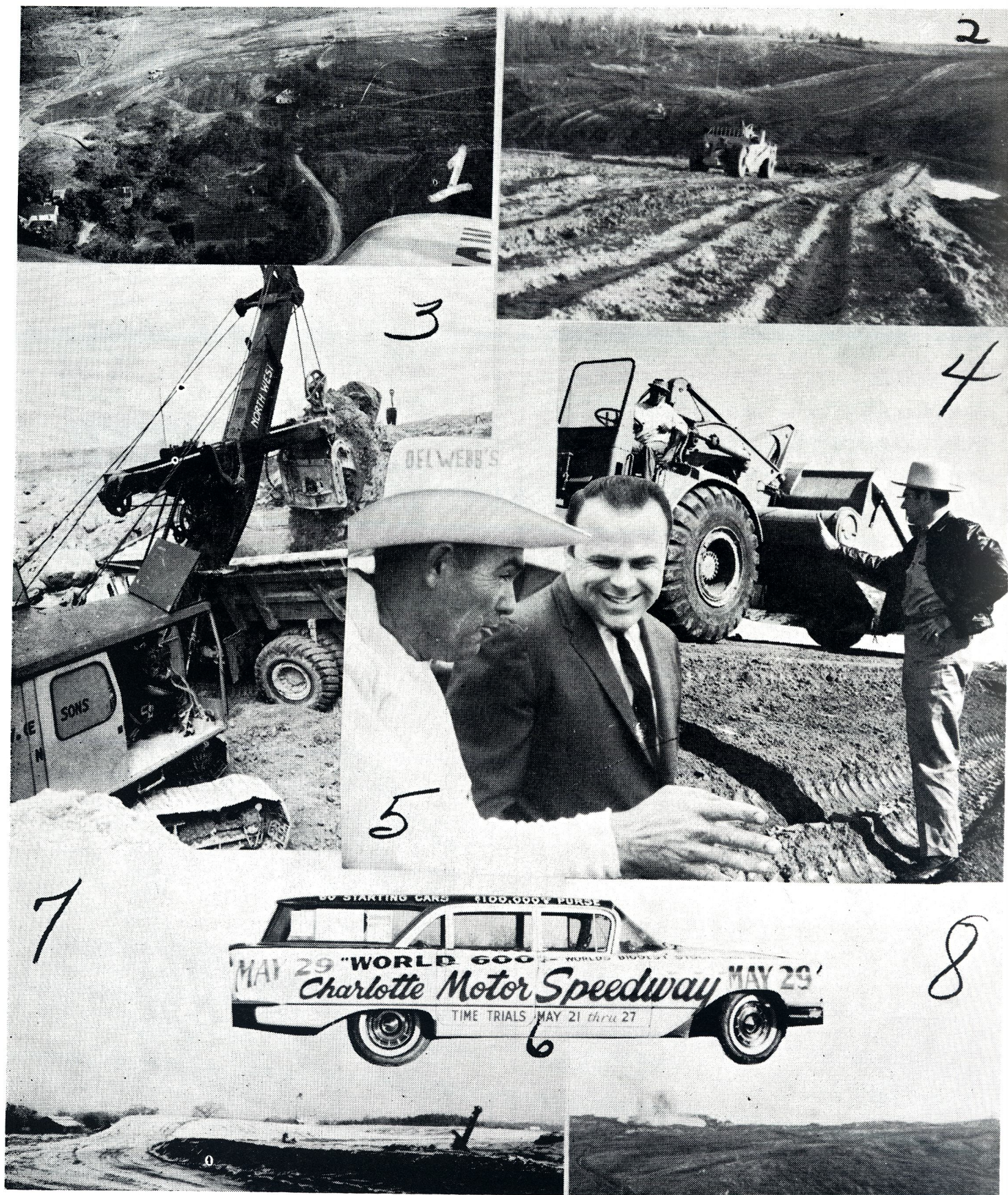
CHARLOTTE MOTOR SPEEDWAY CONSTRUCTION — 1. An aerial view taken in October, 1959 during early stages of construction. The pit area is where the house in the center is shown. 2. Big earth-moving pan works on third turn. 3. Big shovel pours dirt into back of back-dump truck. This scene was repeated 24 hours a day on many, many occasions. 4. Curtis Turner holds his hand up to give you an idea of the 24-degree elevation of the turns. 5. General Manager Bruton Smith (right) talks to veteran NASCAR driver Jimmy Thompson during a visit to the Speedway. 6. Here's one of the 1960 Buick Station Wagons used by Charlotte Motor Speedway. They've been most dependable, economical and comfortable on the tours they've been taken around the country. 7. The scene after one of three big winter snows that crippled construction progress. 8. The mushroom in the background came up when crews dynamited some of the rock near the second turn.
