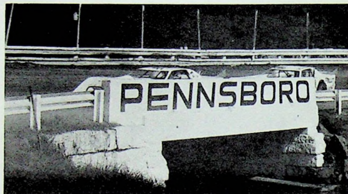
Pennsboro Bridge (Newkirk)
